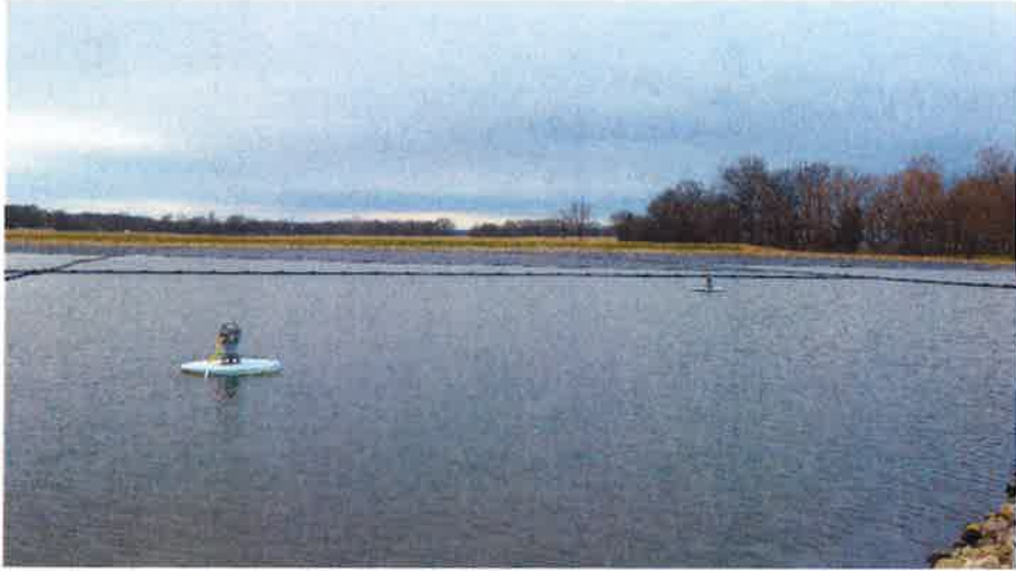
Aerators in Lagoon 3 Looking west at Lagoon 3
