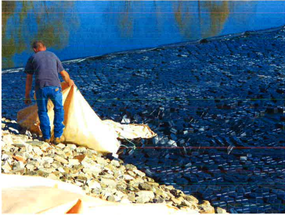
Installing HexProtect Tiles
