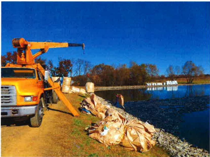
Installing Tiles Looking north along the west bank of Lagoon 3
