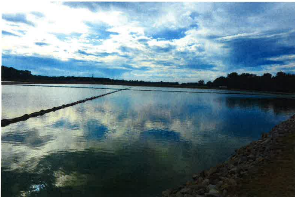
Baffles and Booms in Lagoon 3 A second view looking west
