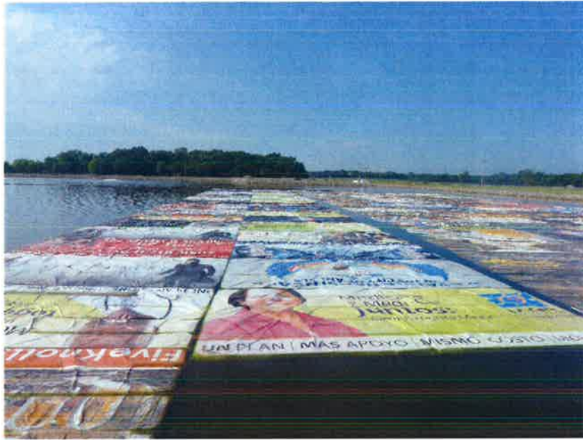
Covers Deployed over Lagoon 2 Looking South
