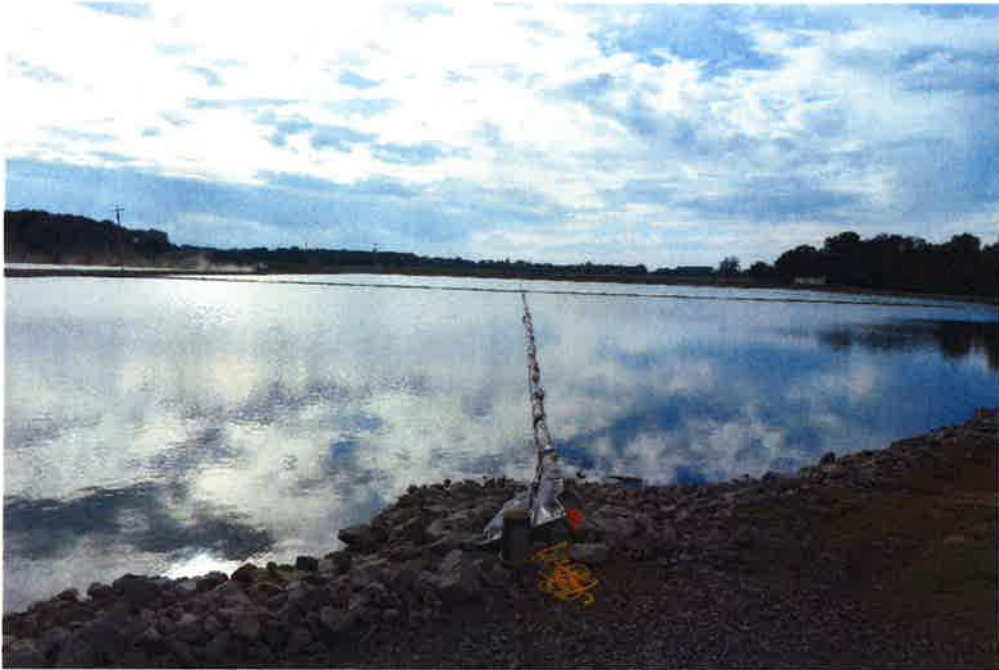
Baffles and Booms in Lagoon 3 Looking West
